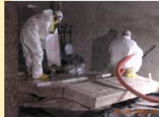
The walls, floor and ceiling of the "Infinity Room" were cut into blocks for shipment to a radioactive waste disposal site.
