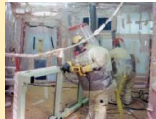
Workers were required to wear cumbersome protective clothing while dismantling equipment.
