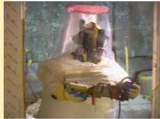
A worker removes an old, abandoned jackhammer from the "Infinity Room."
