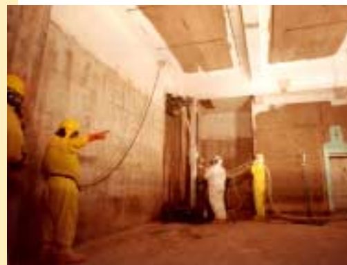
Workers use ultra high pressure water jets to decontaminate the structure.
