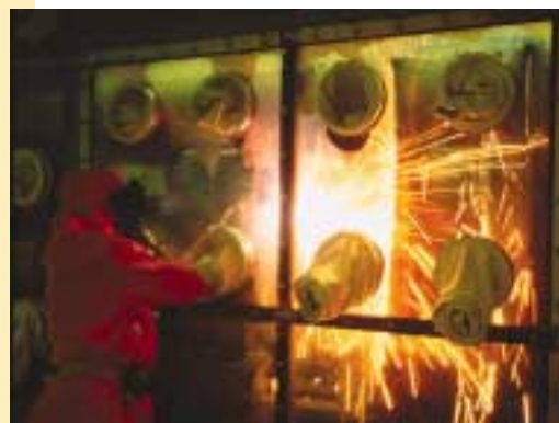
Using plasma-arc torches to cut up stainless steel gloveboxes significantly improved safety.
