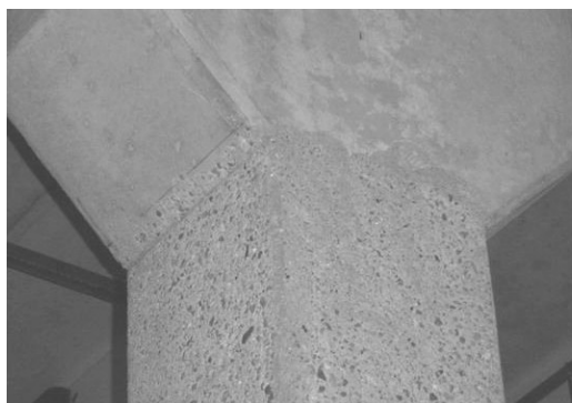
Figure 7. Hydrolased Concrete Columns
